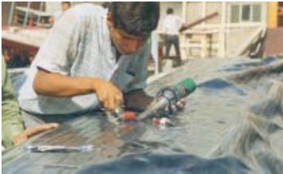
Hot Air Welding
