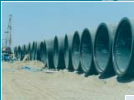
HDPE T-GRIP™ lined pipes on SPC, U.A.E.
