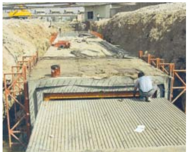
KST Liner on form. Culvert construction, Mosul, Iraq
