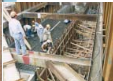
Construction of T-GRIP™ PVC lined culvert
