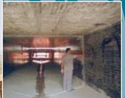
Finished Culvert, Iraq
