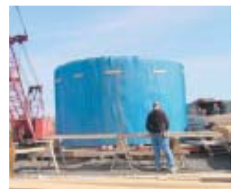
Digester Dome construction with blue polyethylene T-GRIP™ lining in U.S.A.
