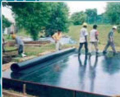
Liner preparation, Singapore
