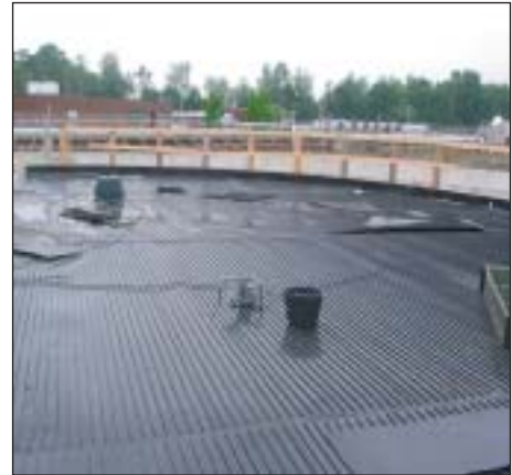
Soffit of wastewater tank structure
